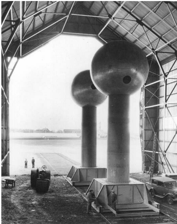
THE GENERATOR IN THE HANGAR AT ROUND HILL
