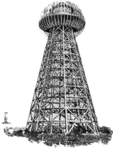
Fig. 6. A tower used by Tesla to transmit wireless signals. He also hoped to use such a tower to transmit large amounts of electrical power over long distances.
