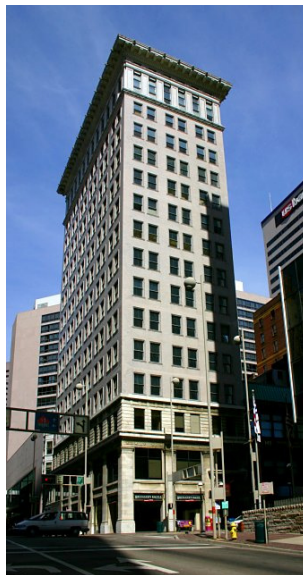
Fig. 1.1 The Ingalls Building built in 1903 in Cincinnati, Ohio [15].
