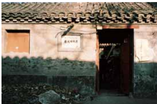
Former residence of Cai Yuanpei after repairs
