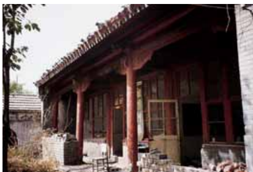
New Guangdong Guild Hall before demolition, (photo by Wang Jun, September 18, 1998).
