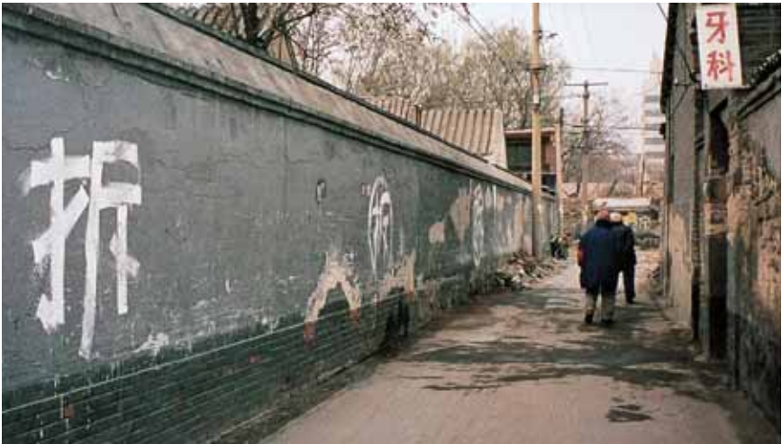
Jing'er Hutong about to be demolished. Note the Chinese character chai (to be demolished) on the wall, (photo by Wang Jun, November 23, 2000)
